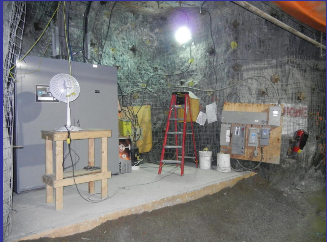
Underground Monitoring Area for Test Freeze
