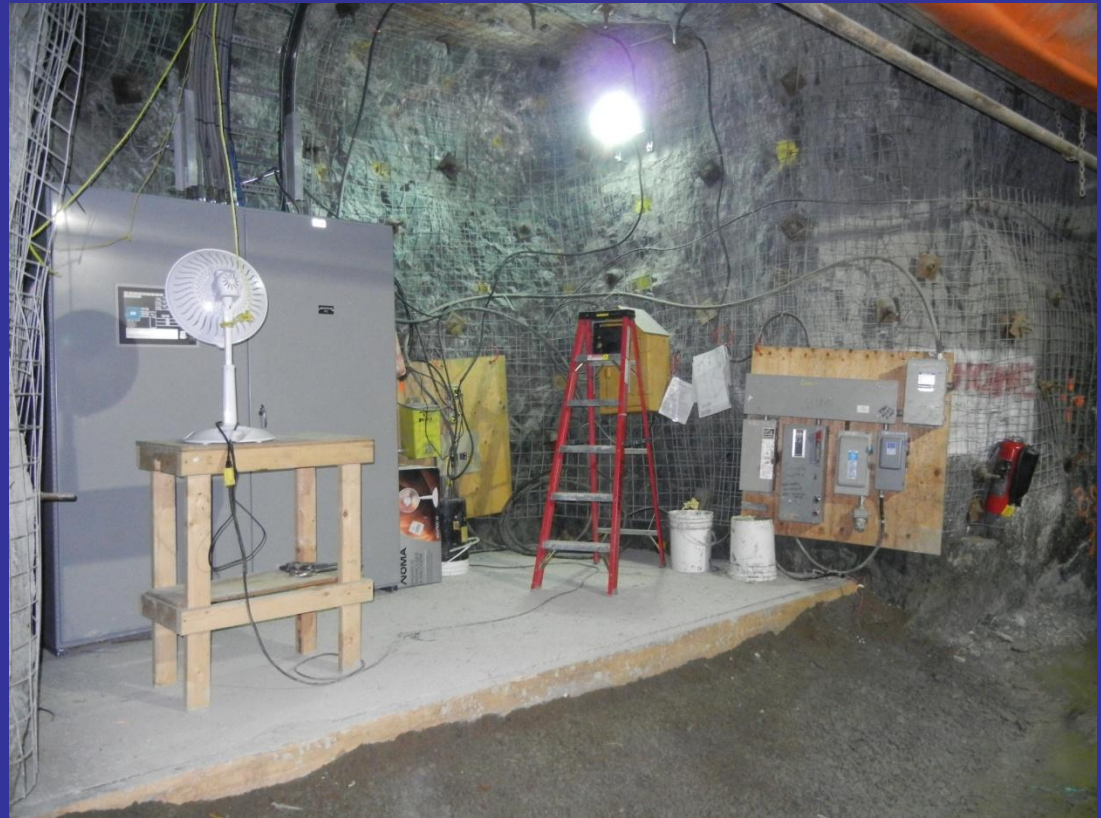
Underground Monitoring Area for Test Freeze
